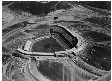
A birds-eye view of the Dodger Stadium construction and terraced parking at Chavez Ravine.
