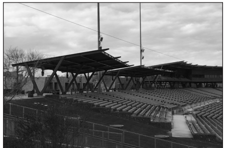
In 2018, two new 100' shade structures were added on the first-base concourse to enhance the fan experience.
