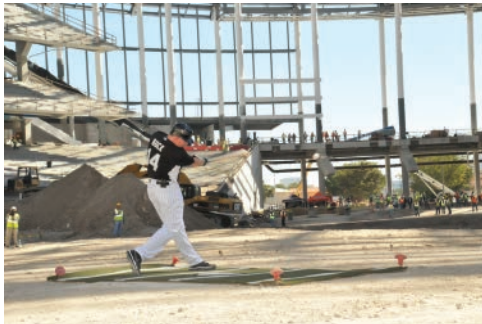
Marlins players take batting practice at Marlins Park in front of construction workers and media.
