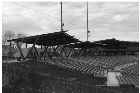
In 2018, two new 100' shade structures were added on the first-base concourse to enhance the fan experience.
