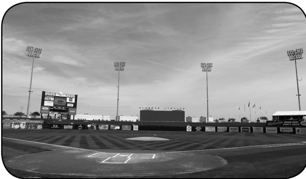
SURPRISE STADIUM - SURPRISE, ARIZONA
