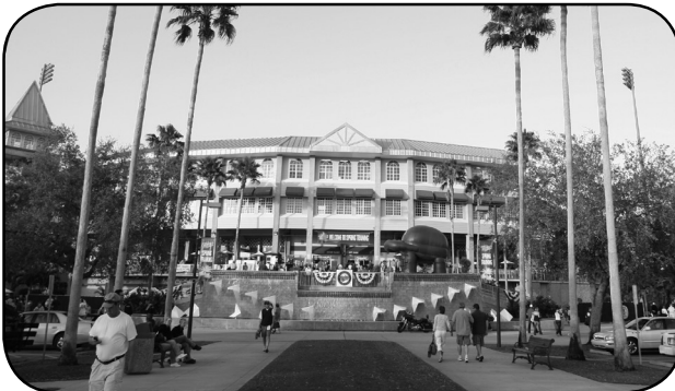
HAMMOND STADIUM - LEE COUNTY, FLORIDA
