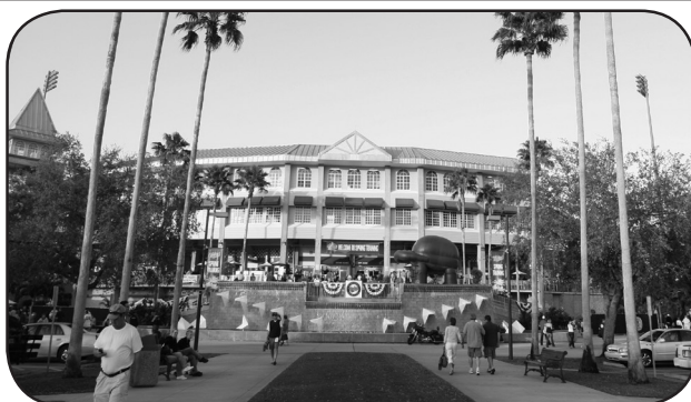
HAMMOND STADIUM - LEE COUNTY, FLORIDA
